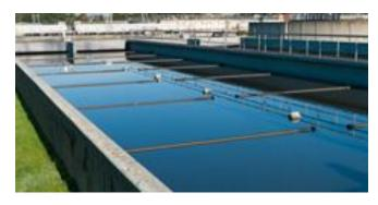
approximately 6,850 customers in and around Gaffney. The Board operates two wastewater treatment plants. The Clary Plant can treat 3.6 million gallons per day; and the Broad River Plant treats 3.5 million gallons per day. An expansion of the Broad River plant to a capacity of 4.0 million
