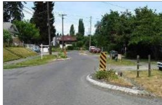
Chicanes require all vehicles to reduce their speeds.
