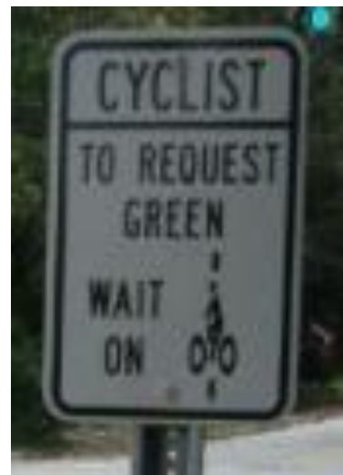
Figure 7-7: Example of existing bicycle detection symbol in Greenville
