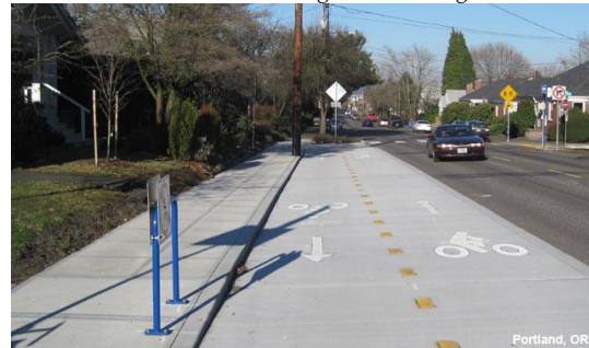
Recommended Design – Two-Way Cycletrack
