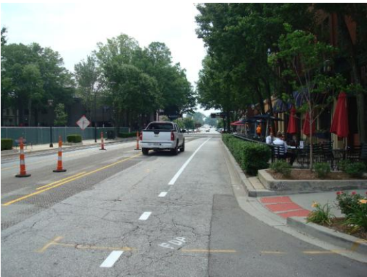
West Washington Street in Greenville was re-stripped to convert four vehicle travel lanes into three travel lanes with bike lanes.
