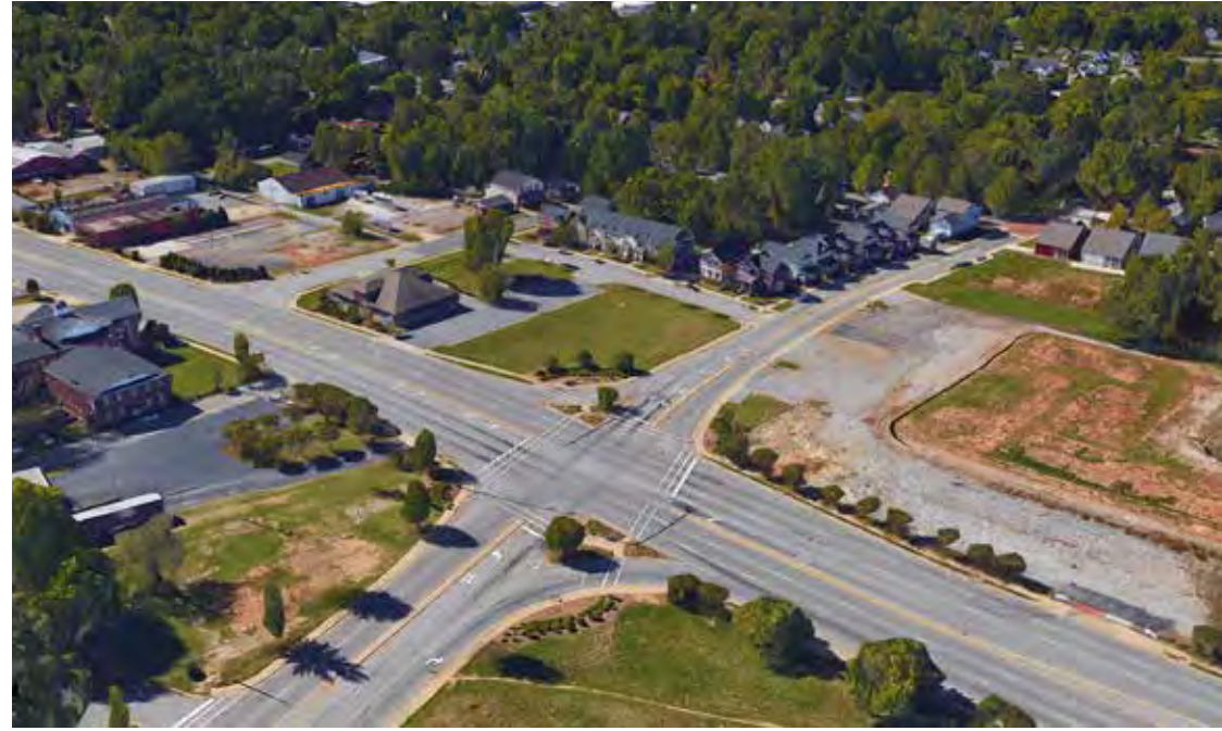
Aerial photograph of existing Pete Hollis and Stone intersection
