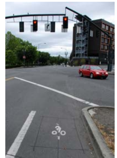
Bicycle-activated loop detector and pavement marking.
