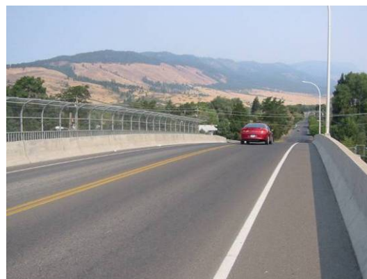
Facilities such as roadway shoulders accommodate bicycle travel and provide a safe location for disabled vehicles to stop
