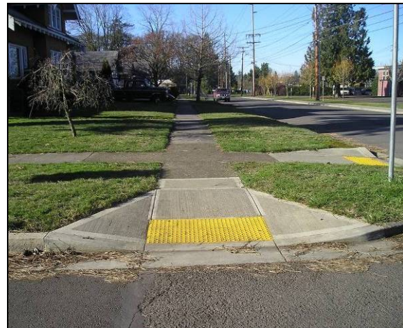
Example of an ADA-compliant perpendicular curb ramp with a raised tactile strip
