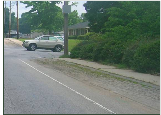
Overgrown sidewalk next to asphalt ditch at Brushy Creek/Pearson
