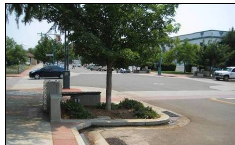
Curb bulb-outs can include street trees
