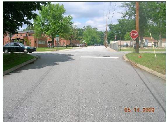
Lack of sidewalks on 2 nd Avenue one block away from East End Elementary
