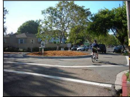
Traffic calming circles are attractive treatments for shared roadways
