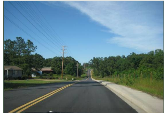
New sidewalk along one side of Wimberly Lane
