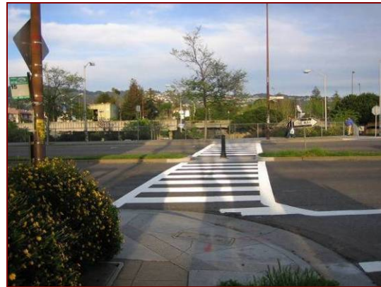
Ladder pavement markings are the preferred crosswalk design for Easley
