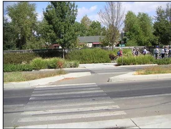
At-grade crossings can be made safer and easier with pavement markings, pedestrian refuge islands, and other treatments
