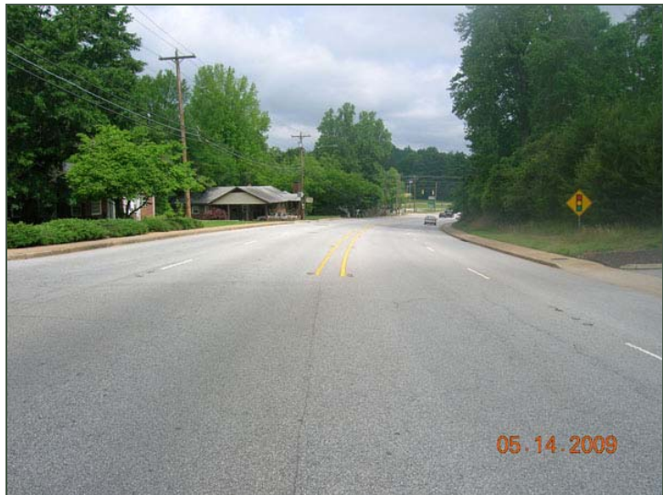
Existing Conditions along SC 135 northbound approaching Fleetwood: 4 lanes, undivided.
