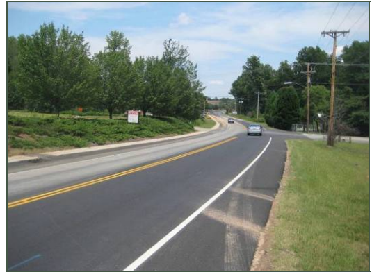
Fleetwood Avenue near the Hospital was recently repaved and restriped to include a shoulder bikeway
