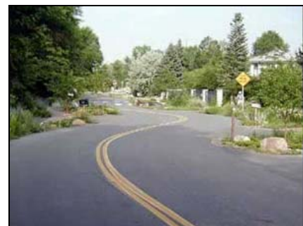
Chicanes can be used on shared streets to reduce traffic speeds
