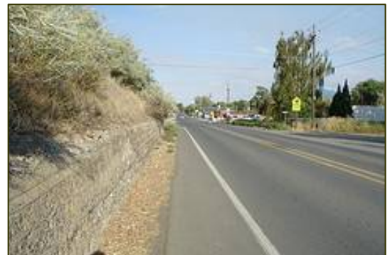
Example of a four-foot shoulder bikeway
