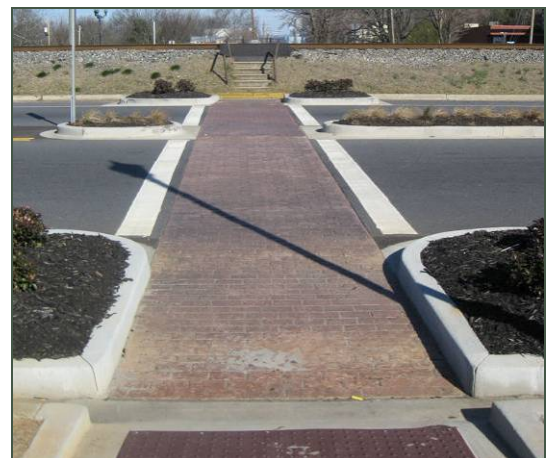
High-quality pedestrian crossing with ADA ramps, visible cross-walk, and pedestrian refuge on Main St
