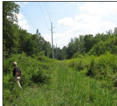
Utility corridor in Easley that could provide space for future trail
