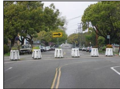
Traffic diverters allow bicycle and pedestrian traffic to go through, while blocking automobiles
