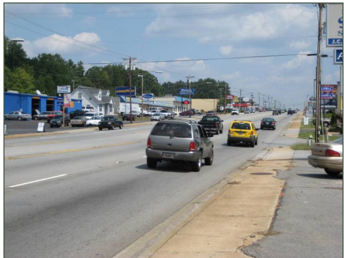
Existing conditions along SC123: Deteriorated and uncomfortable pedestrian infrastructure along with traffic, land use and streetscape patterns that create a hostile environment for pedestrians and cyclists.
