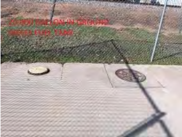
Diesel UST (20,000 gallon) fill port and manhole
