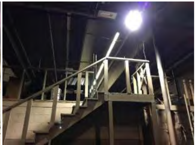
Stairs leading to storage space above offices
