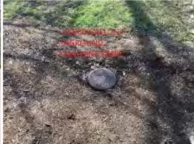
Gasoline UST (10,000 gallon) fill port
