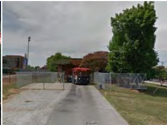
View of fueling canopy from street
