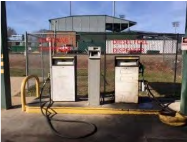
Gasoline dispenser Fuel management system Diesel dispenser
