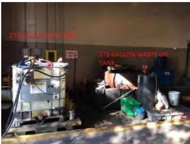
DEF Tank (275 gallon) Waste Oil Tank (275 gallon)
