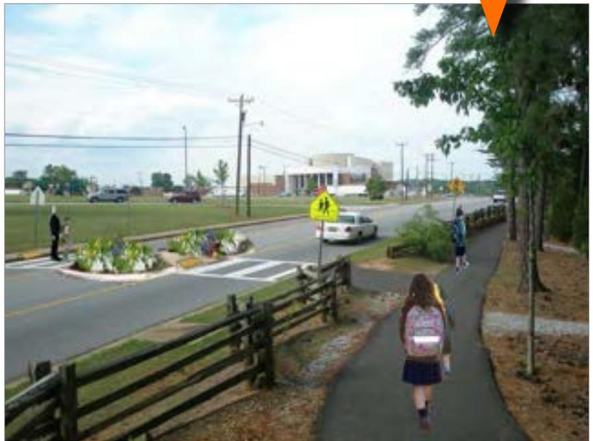
The intersection of SC 290 and SC 296 is very dangerous for pedestrians. Wide turning radii and long crossing distances make it difficult to navigate for pedestrians. Reducing the curb radius, adding a median refuge island, making the crosswalk more visible, and improving the pork chop island would improve this intersection dramatically.
