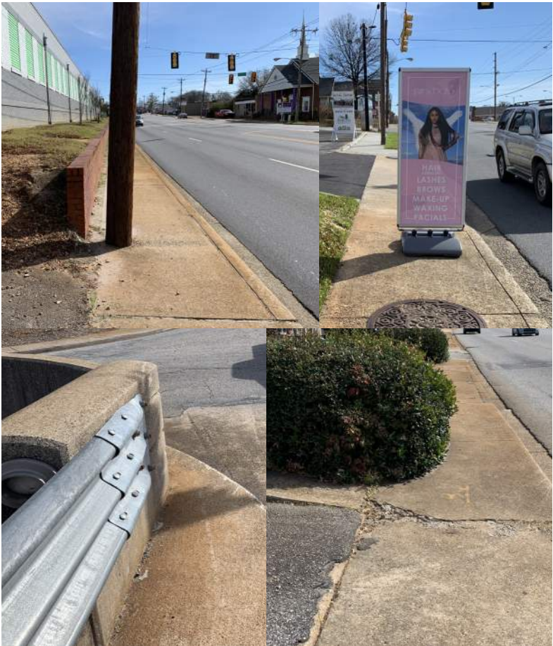
Existing conditions along Laurens Road with utility poles, signs, and vegetation impeding on the narrow sidewalk, as well as sidewalks that dead end
