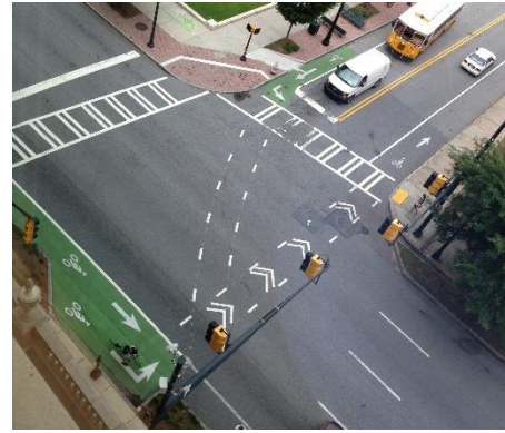
Bicycle Intersection Pavement Markings
