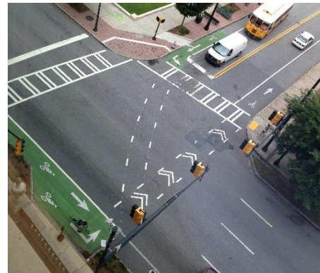
Bicycle Intersection Pavement Markings
