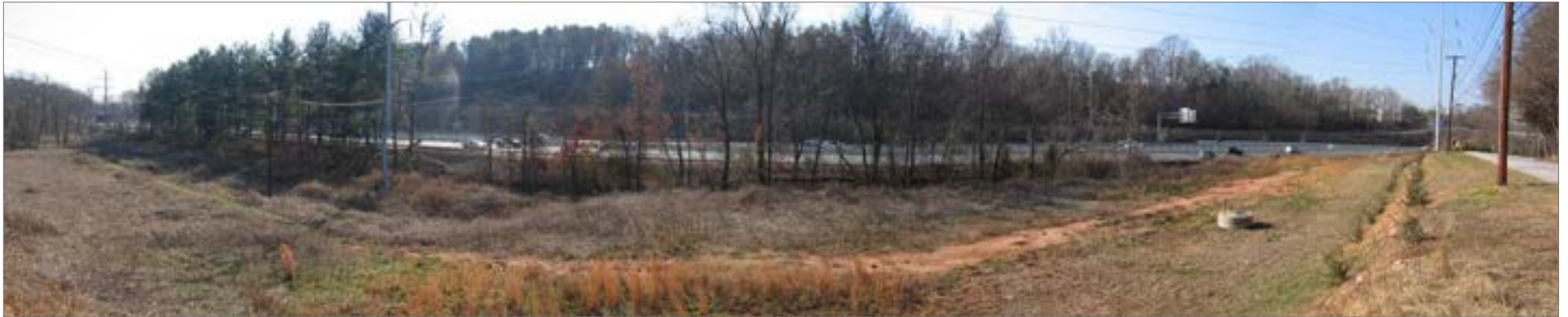
Existing Conditions: Sewer corridor along the north side of I-385, near Lowndes Hill Road
