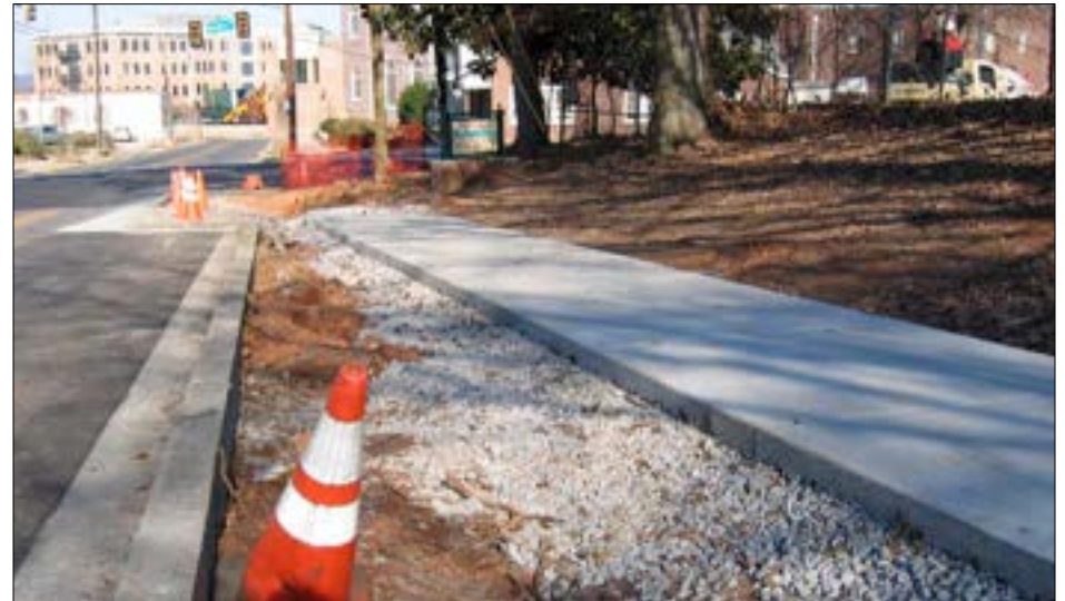
Sidewalk construction on Green Avenue
