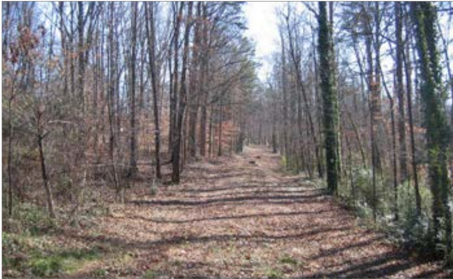
Existing Conditions: Sewer easement along Brushy Creek, near Pacific Ave.
