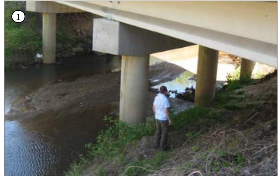
I-85 bridge over Brushy Creek.
