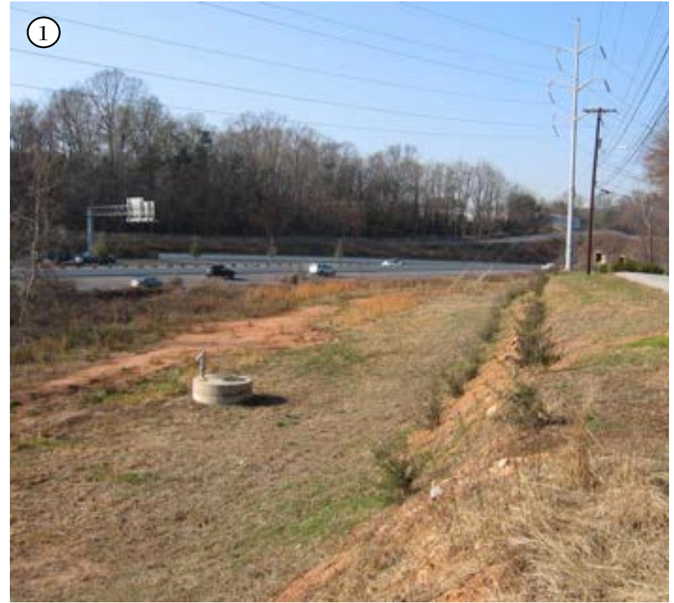
Sewer and power line easement along Lowndes Hill Road (looking west).
