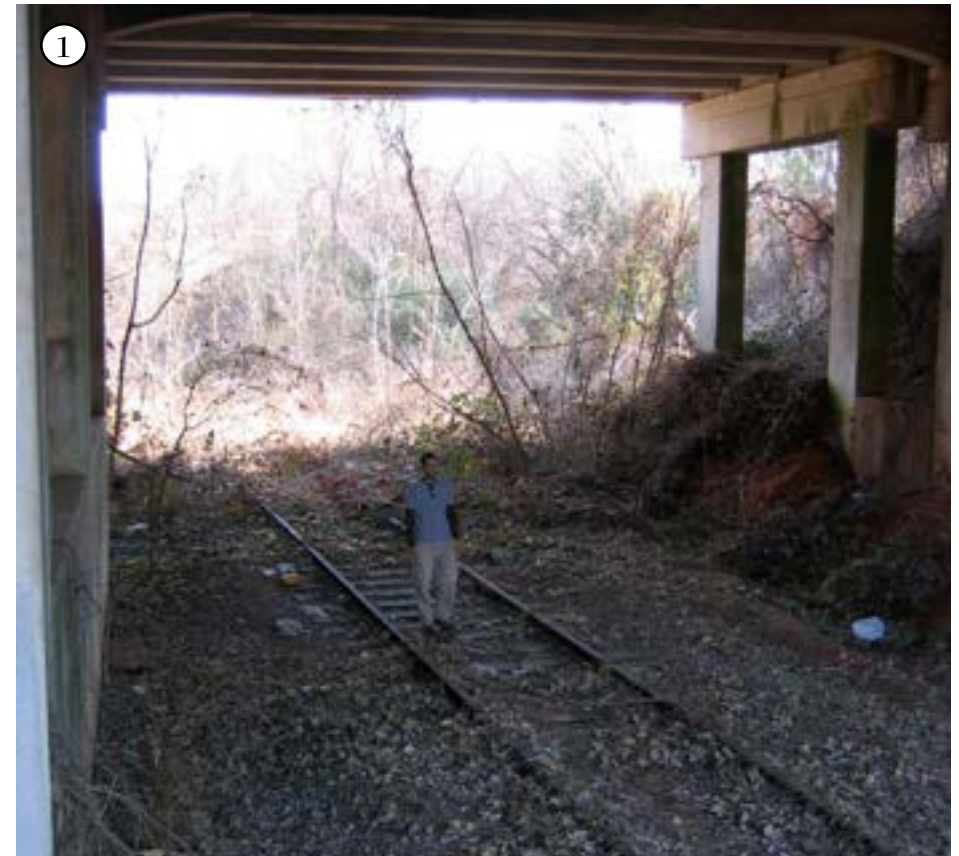
Clearance underneath the Pleasantburg Road bridge.
