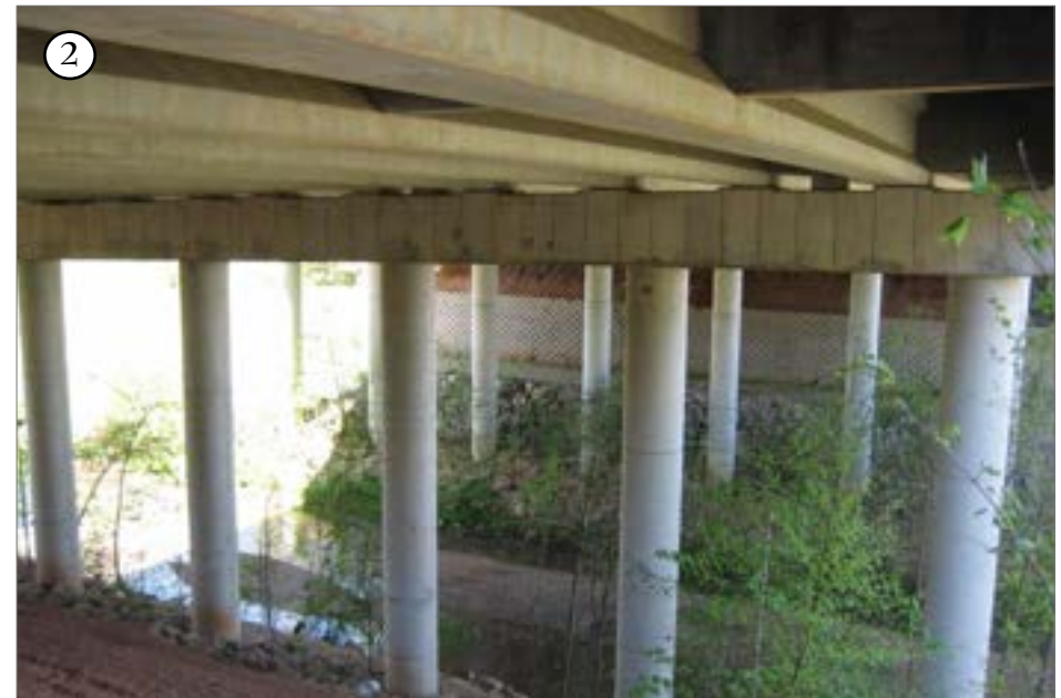
S. Pleasant burg Drive Bridge over Brushy Creek.
