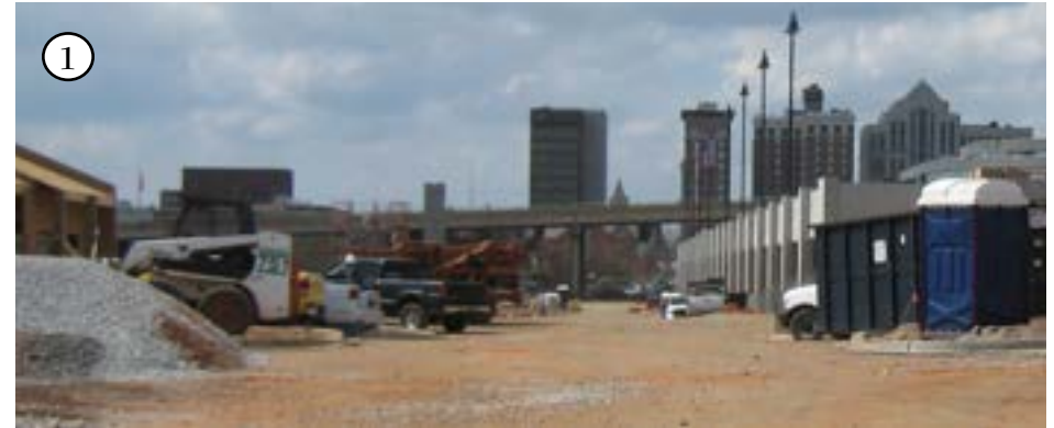
McBee Station under construction along the proposed corridor.
