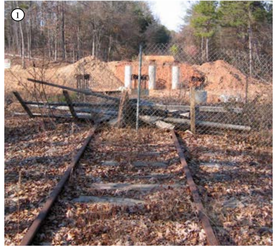
Rail corridor at Woodruff Road, looking north at new bridge construction.
