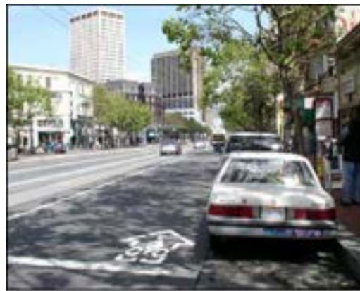
Sharrow installed on Market Street, San Francisco
