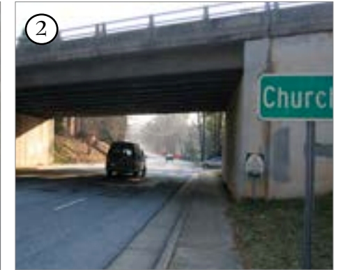
Church St. underpass with sidewalk.
