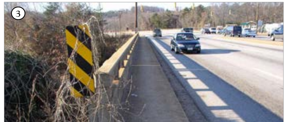
Sidewalk along the Pleasantburg Road bridge, over the rail corridor.
