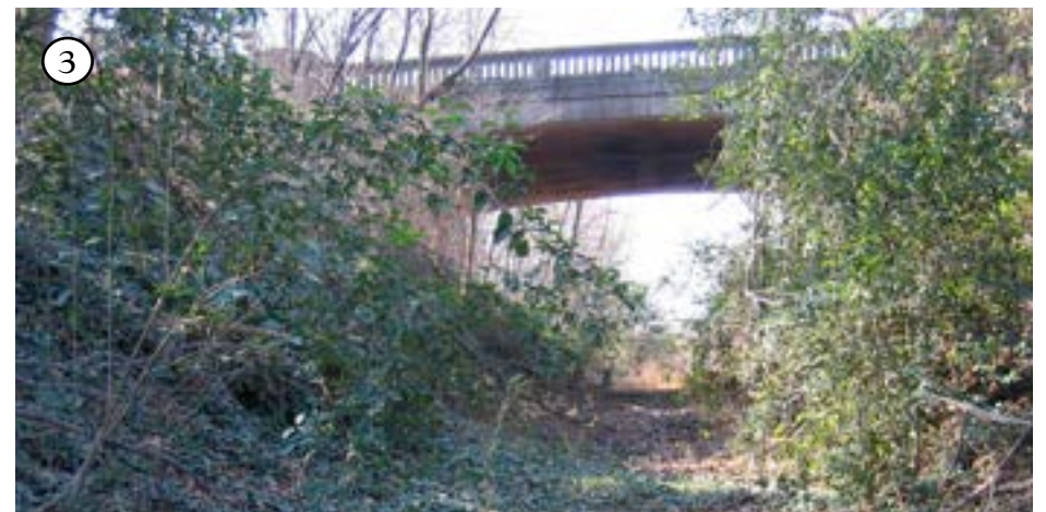
McDaniel Avenue bridge over abandoned rail/future trail corridor.
