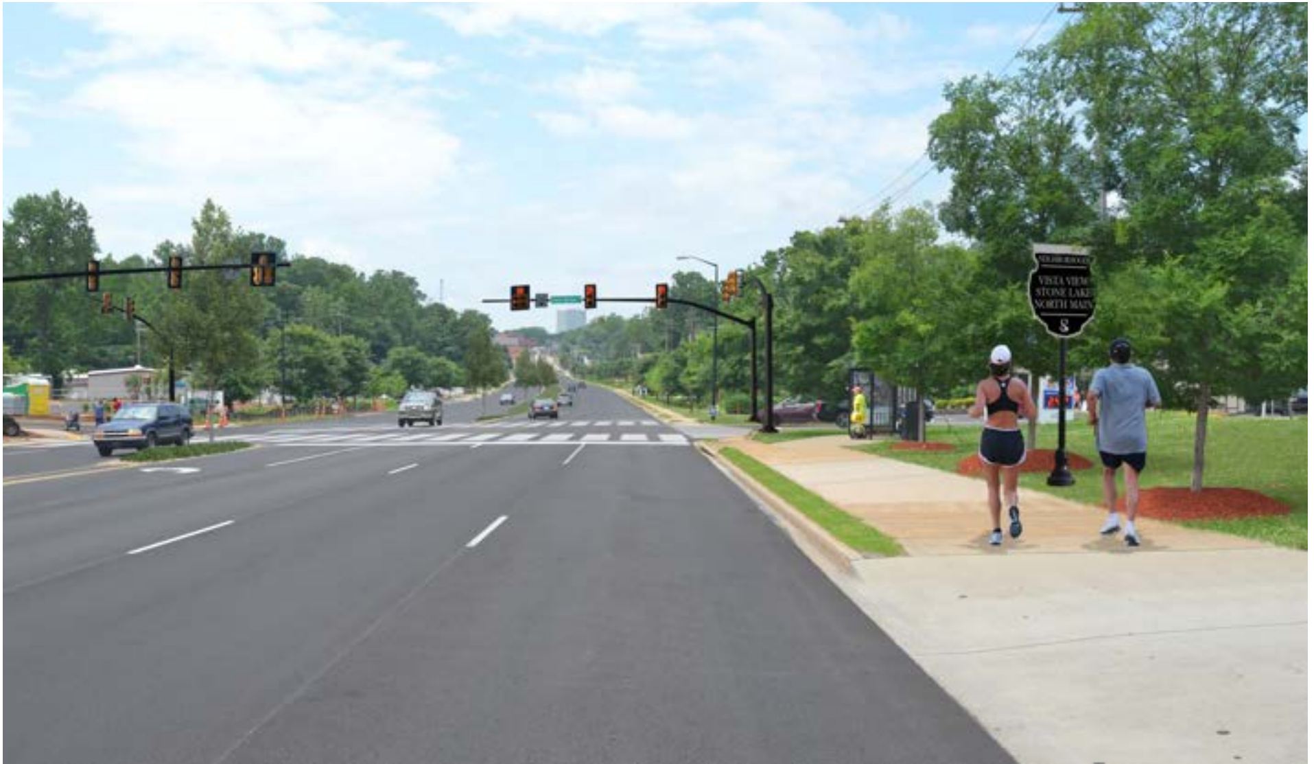
Proposed conditions of Wade Hampton Boulevard at the intersection of Chick Springs Road showing multi-use path, mast-arm traffic signals, additional tree plantings, narrowed curb cuts, neighborhood demarcation signs, and center landscaping.
