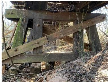
Figure 6: Timber Frame with Timber Mud Sill
