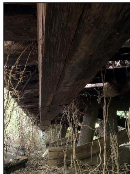
Figure 3: Portion of Superstructure Slid off Cap
