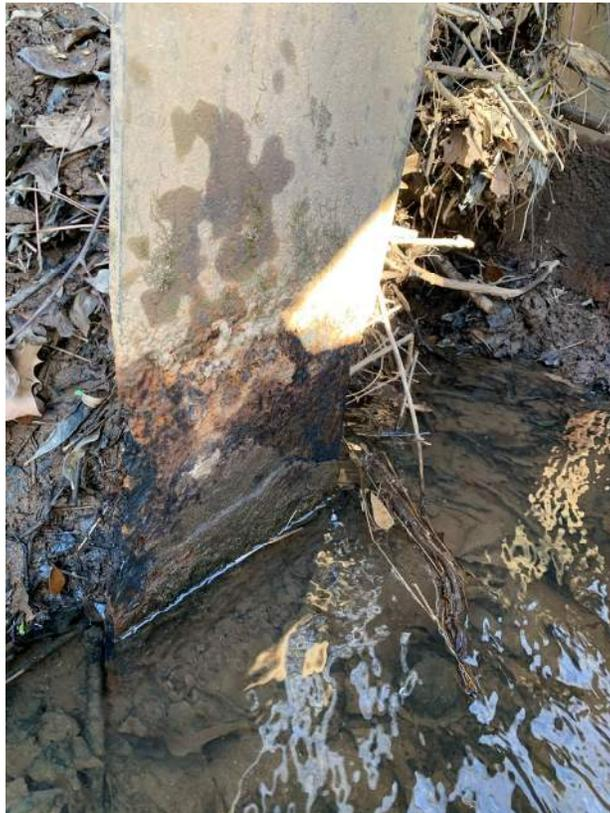
Bent 17-2 (Pile Decay at Mudline)
