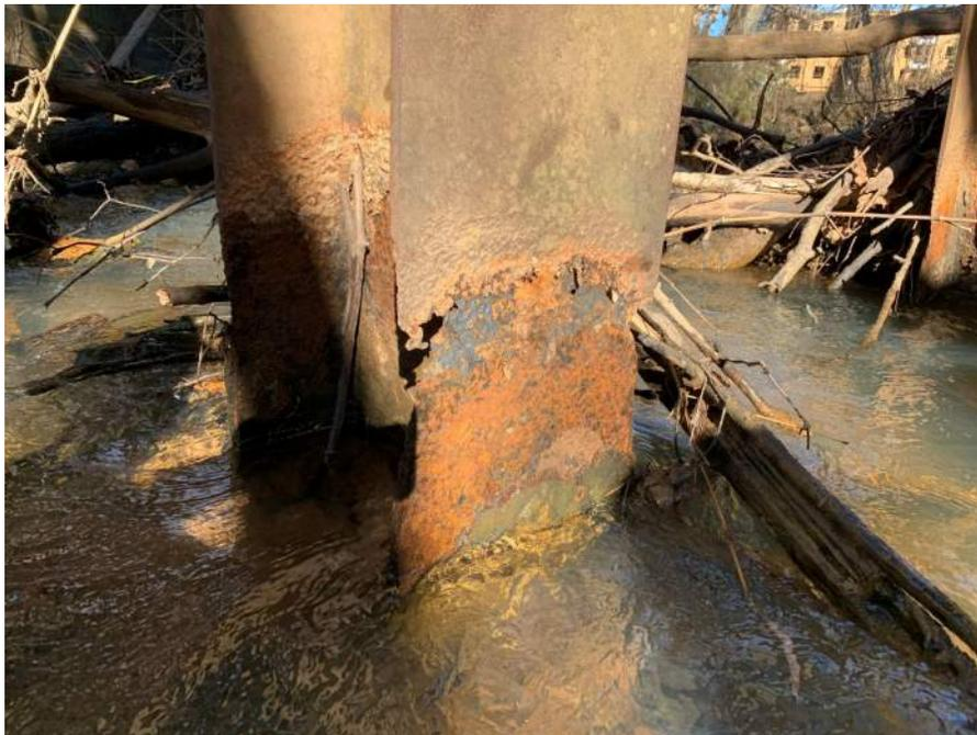
Bent 19 (Pile Deterioration)
