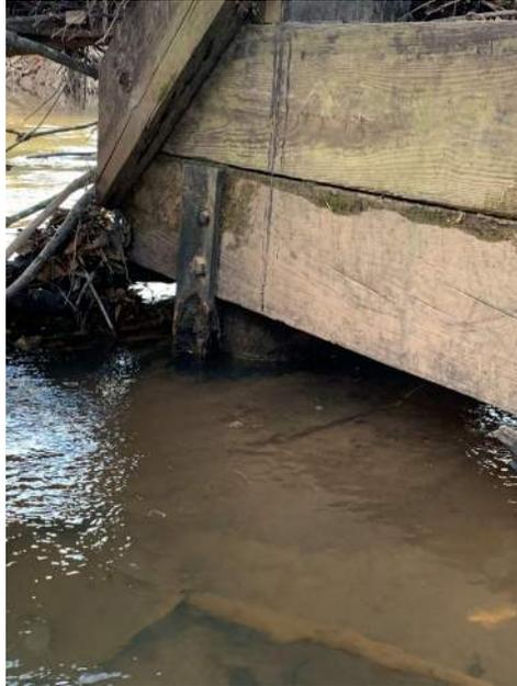
Bent 17-1 (Motor Grader Blade Repair for Timber Piles)
