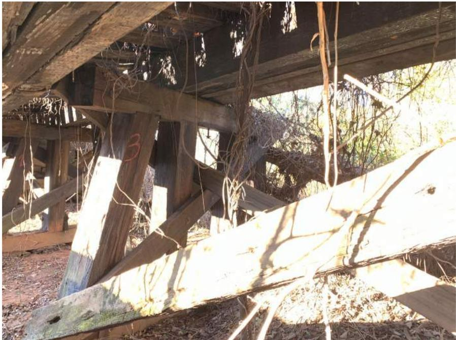
Bent 3 (Displaying Tilting and Torqueing)
