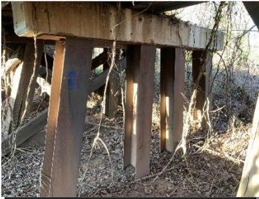
Figure 5: Concrete Cap with Steel Piles
